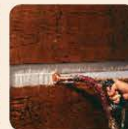
3. Gun Log Jam® over the backer material.
