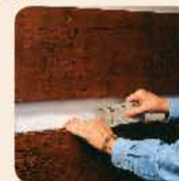
2. Tape the entire joint using polyester tape.
