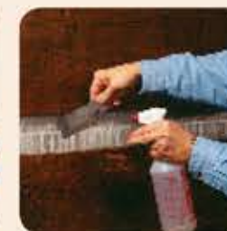
4. Lightly mist the trowel as needed.
