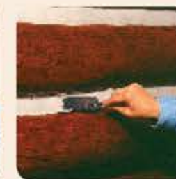
5. Tool to ensure a tight seal to the top and bottom of the chink line.
