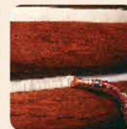
3. Gun Log Jam® over the backer rod.
