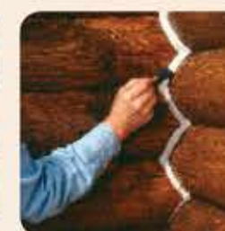
4. Tool to ensure a tight seal.
