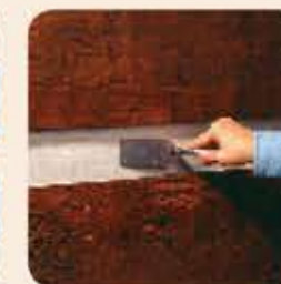
5. Tool to ensure a tight seal to the top and bottom of the chink line.
