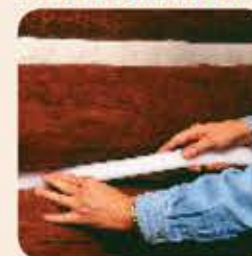
1. Start with logs that are stained with a coating compatible to Log Jam® and have properly installed backer material.
