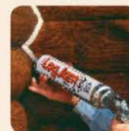
2. Gun Log Jam® over the backer rod.
