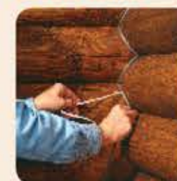
1. Install backer rod into corners of clean, stained logs.
